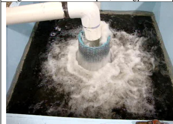
Figure 6. Drain holes open, 75 gpm/tile
