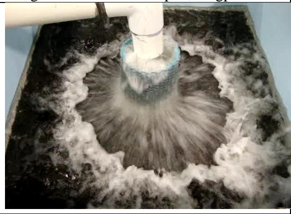
Figure 5. Drain holes open, 62.5 gpm/tile
